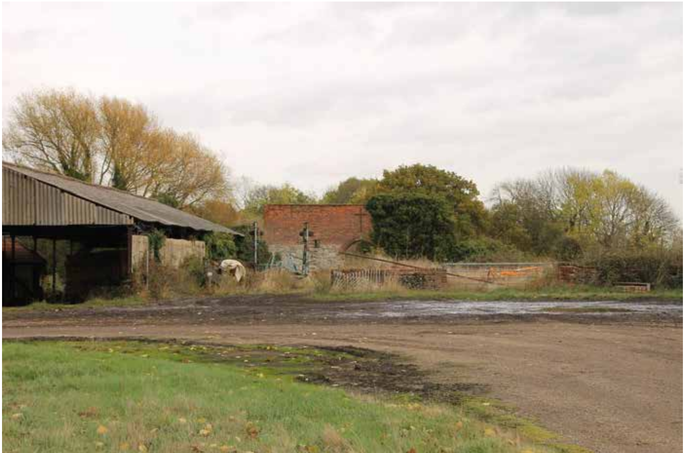
View 2: Looking from the farmyard access road to the gatehouse, the moated site is under the vegetation to the rear of the gatehouse.
